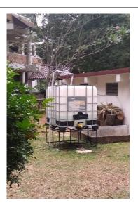
Figure 2. Air conditioning condensation water reservoirs
