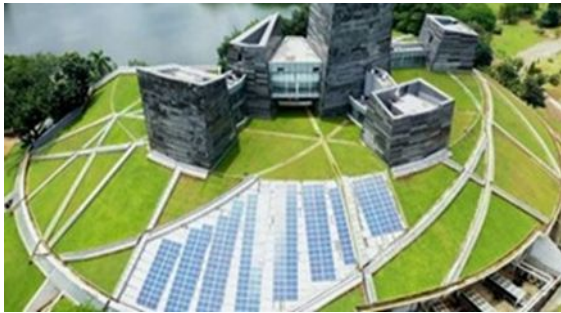
Solar Power Plant On Grid of Library Building
