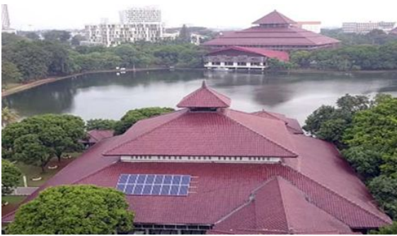
Solar Power Plant of UI Mosque
